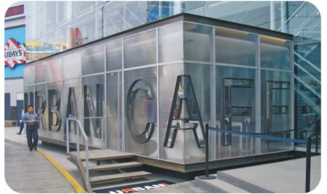
8 mm Clear Sheets, 6-16 Aluminium glazing system
