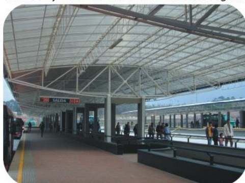
Central Bus Station 10 mm Ice Sheets HCP connecting system
