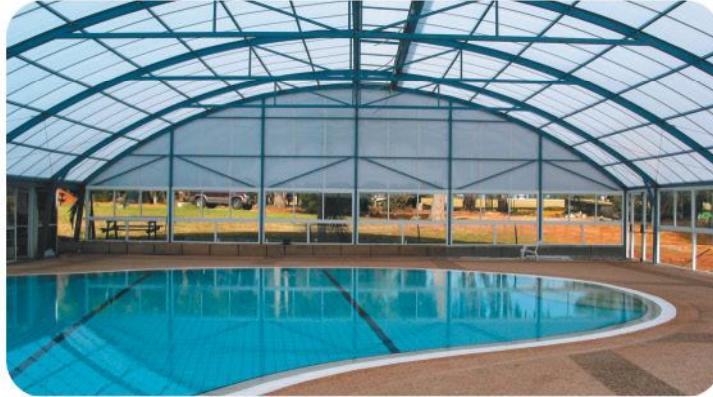
Swimming pool 8 mm Polyshade Silver Sheets, Aluminium glazing system
